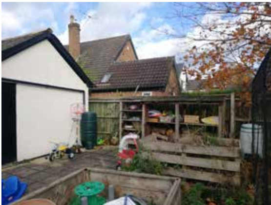
Facing north east, side elevation of no.7
