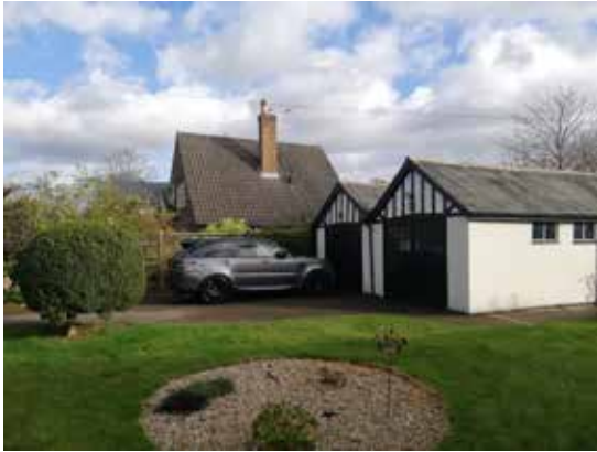
Facing north east, side elevation of no. 7
